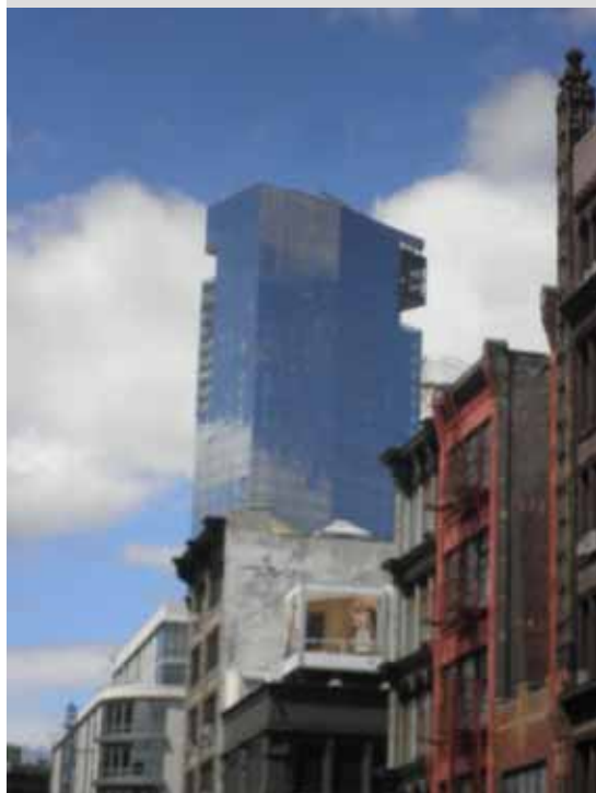
Below: two all glass buildings.
