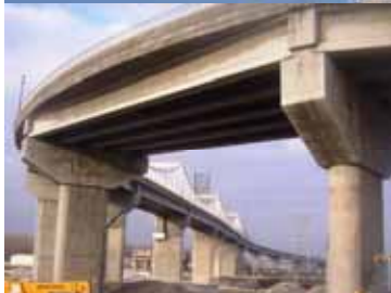
Above: The new bridge over the McAlpine Lock, built by the Corps of Engineers
