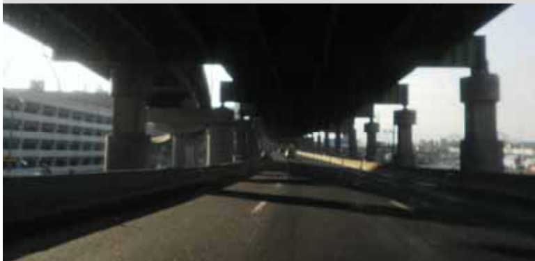
I-64 EB at Mississippi River, St. Louis—Below: I-64 WB
