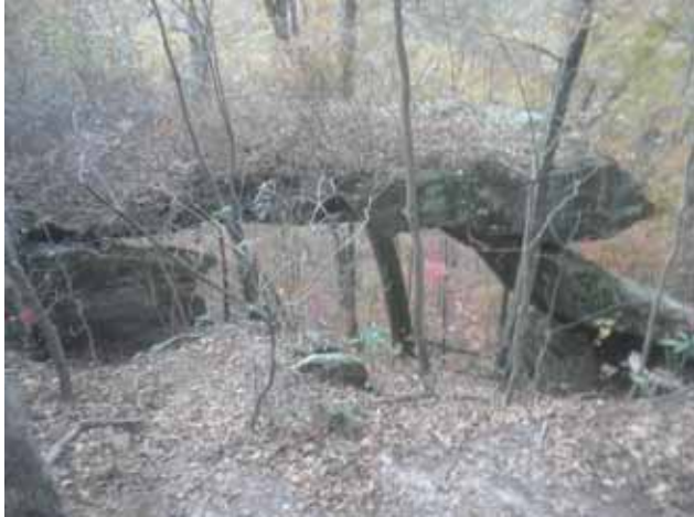
Above: Raven Bridge
