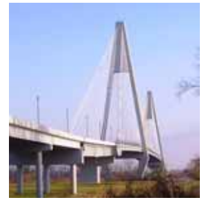
The new Natcher Bridge near Owensboro is a good example of a local access bridge and it cost $55 Million
